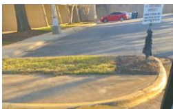
Curb/ sidewalk access at Woodland and West South Street
